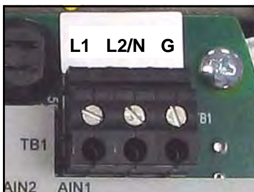
Figure 13: Wiring the AC Line Power
